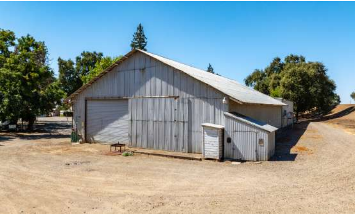
5,600 SF metal roof and cement floor
