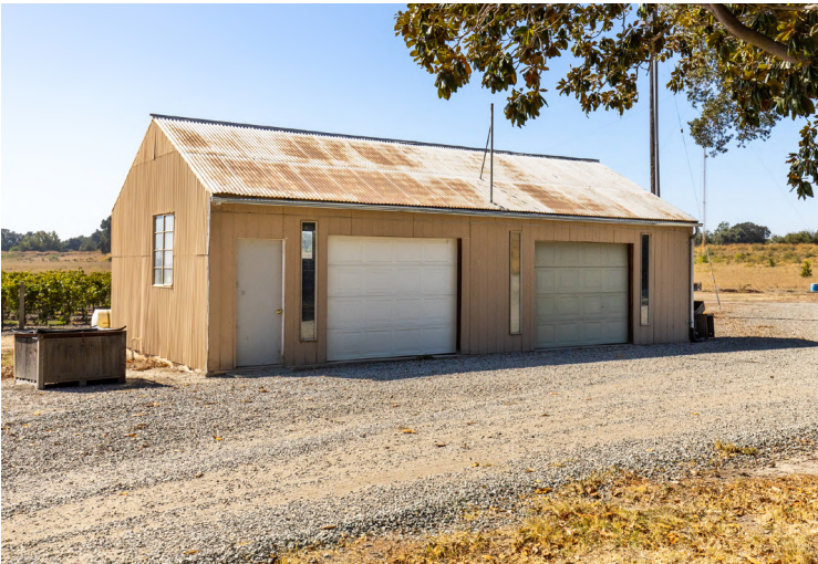
Equipment Storage Shed, 20 x 40-foot wood frame, steel siding/roofing with 8-foot eaves on concrete pad with bathroom and 30-amp 115/230-volt electrical service.
