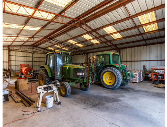
Shop & Storage, 50 x 60-foot steel frame & siding/roofing with 13-foot eaves on concrete pad with 200-amp 115/230-volt electrical service.
