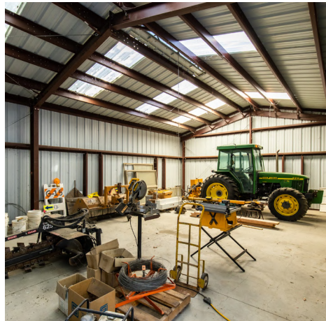
Equipment Storage Shed, 25 x 40-foot, steel frame & siding/roofing, 12-foot eaves on concrete pad. This building also houses the domestic water pumping plant. The domestic water system consists of a 20 GPM centrifugal pump, sediment filters, 120-gal bladder storage and water driven water softener.
