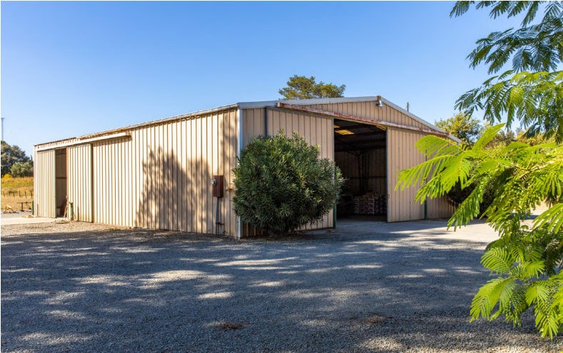
Shop & Storage, 50 x 60-foot steel frame & siding/roofing with 13-foot eaves on concrete pad with 200-amp 115/230-volt electrical service.
