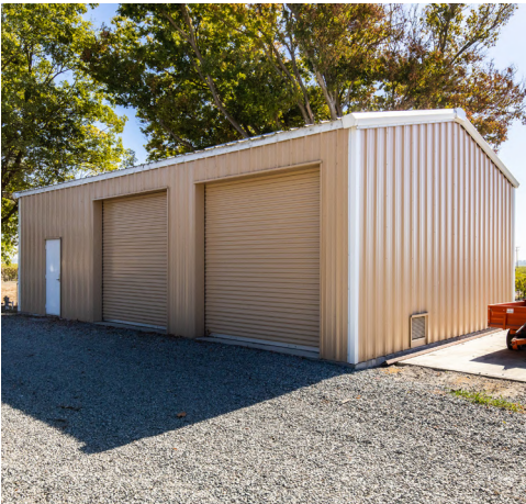
Equipment Storage Shed, 25 x 40-foot, steel frame & siding/roofing, 12-foot eaves on concrete pad. This building also houses the domestic water pumping plant. The domestic water system consists of a 20 GPM centrifugal pump, sediment filters, 120-gal bladder storage and water driven water softener.
