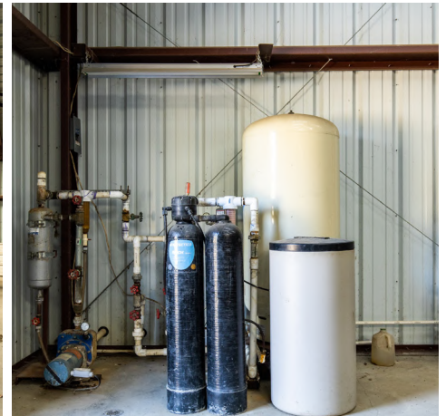
Equipment Storage Shed, 25 x 40-foot, steel frame & siding/roofing, 12-foot eaves on concrete pad. This building also houses the domestic water pumping plant. The domestic water system consists of a 20 GPM centrifugal pump, sediment filters, 120-gal bladder storage and water driven water softener.
